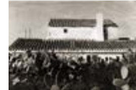
Residential house renovation, Menorca, Spain, 1974, kept by MAO
